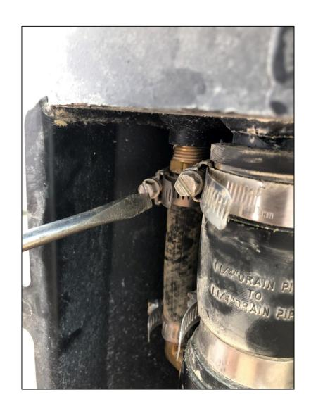
To remove the venturi from the canister you will first loosen the two screw clamps holding the venturi on. Once loose, pull the venturi down. You might have to move it back and forth while pulling down.
